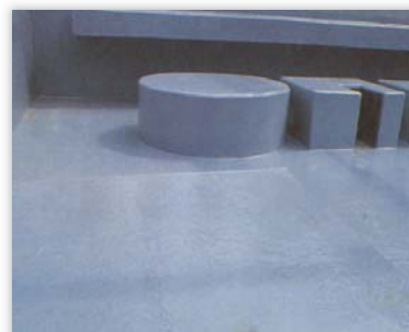
■ FRP LINING FOR WASTE WATER TREATMENT PLANT.
